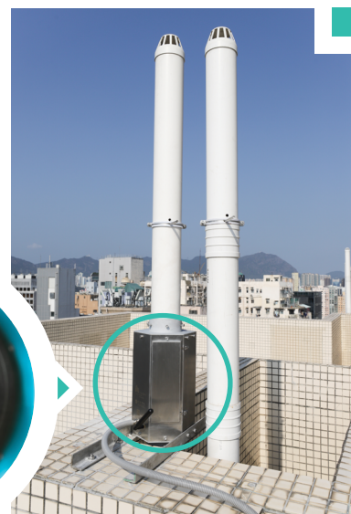
Installing the UV-C VentGuard on the rooftop ventilation pipe of rehousing block at Soy Street.
