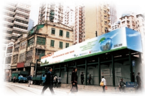
莊士敦道項目的地盤圍板設計融入4Rs 概念。 Hoarding design of Johnston Road project incorporates the 4Rs concept.
