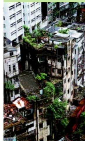
上環皇后街重建項目。 Redevelopment project in Queen Street, Sheung Wan.
